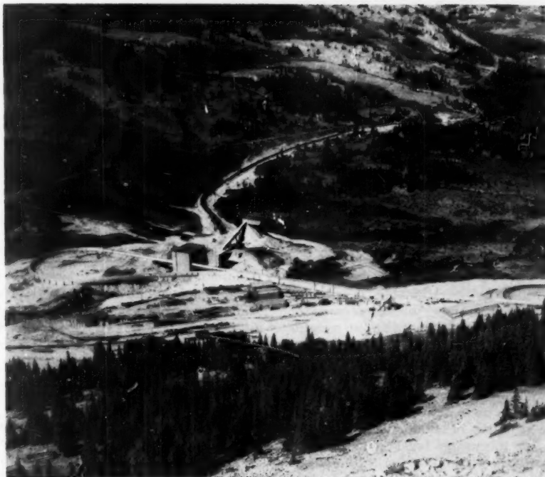
SURFACE facilities for Storke level at Climax mine includes crusher buildings and storage area (center left), connected by covered conveyor system going to mill (out of picture to right). Mine portal is near changehouse (center right).
